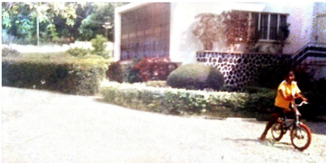
Figure 1: Landscaped building in reserved area of Enugu
