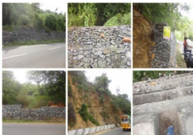
Figure 3: Remedial Actions of Landslide in Nilgiri region
