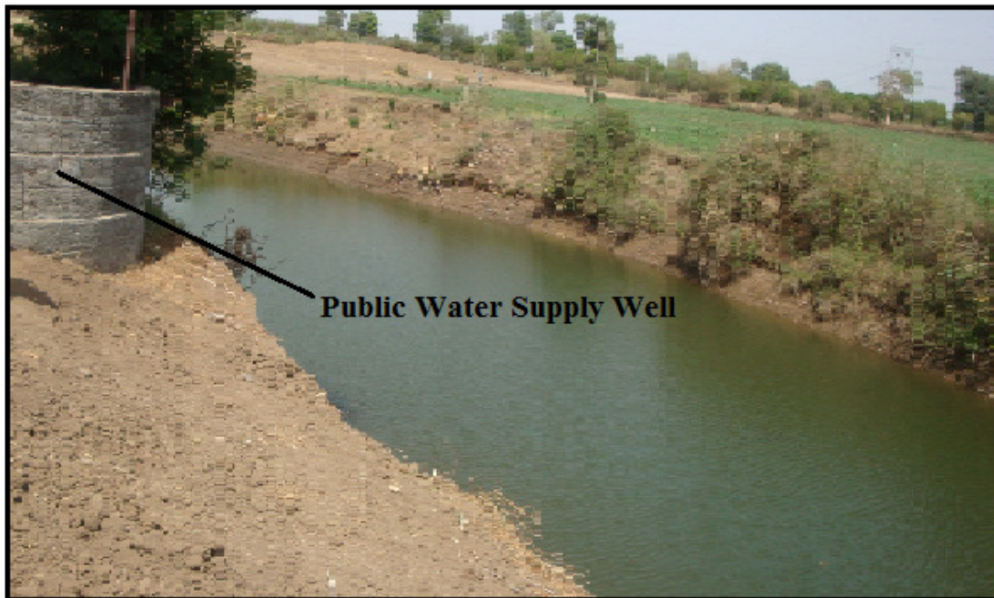
Plate 2: Stored water after nala deepening and widening
