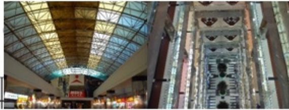
Fig1.2: atrium roof and view of BCSC
