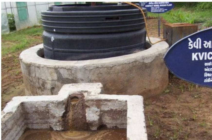
**Fig. 1: KVIC biogas plant**
